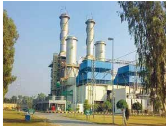
KAPCO Power Plant
